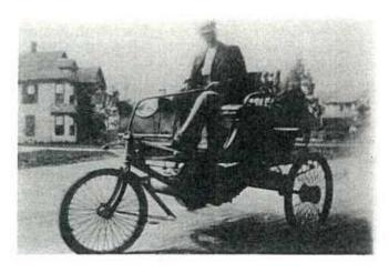
Ray Van Auken on his 1900 Knox which was handed down through the Van Auken family. The machine ran on a 1 cylinder, air-cooled engine. On its tubeless front pneumatic tire and two  $2.50 \times 24$  solid tires the three-wheeler could reach 8 mph when the throttle was opened wide.
