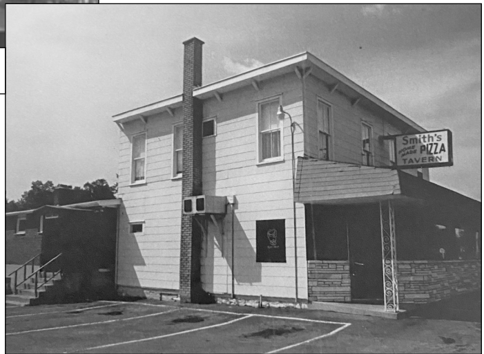
Photo 1990 includes dining room addition on the back and from porch enclosure.
