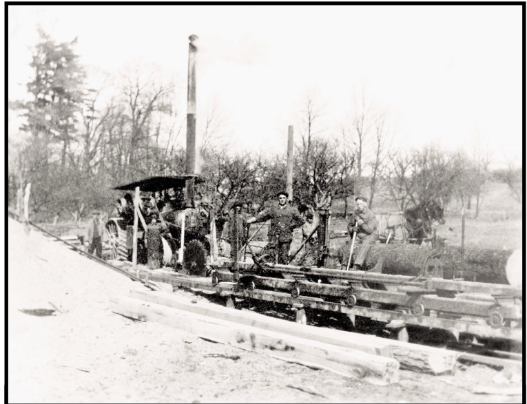
Sawing the lumber into the boards and other pieces needed to build the new barn replacing the old one that was destroyed by fire in 1915 .
