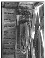
ed in the peaks of the barn roofs. They were attached to a pulley system with ropes. A horse, and later a tractor, would move forward to pick up the hay and then would back up to lower it. This photo shows a hay fork from Jim Slingerland's farm.
