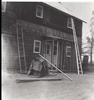
Barn converted into the Le Vie home in 1952
