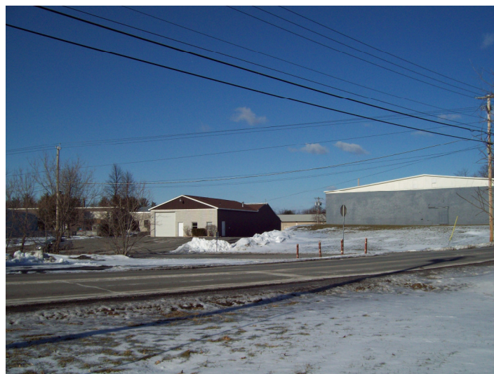
Same site as it appears today.
