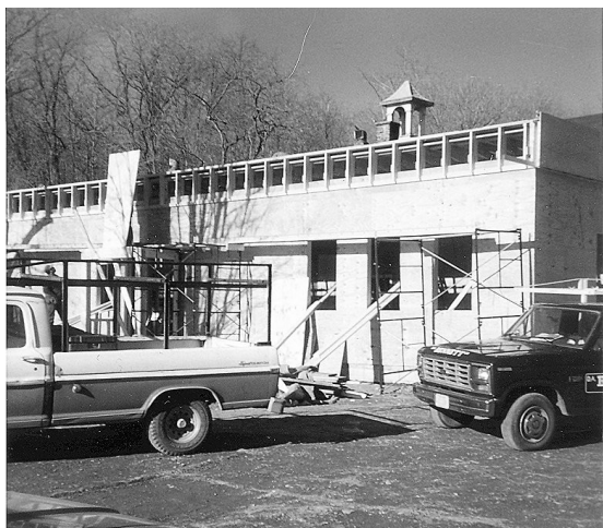
Construction began in October 1988
